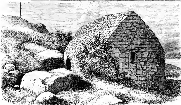
Fig. 13. Oratory on Inchcolm, as lately repaired by the Earl of Moray.
